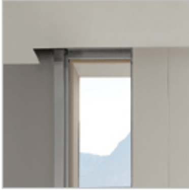
Line flush with the ceiling
